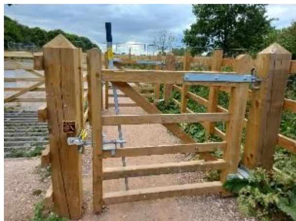
Photo 3. Airlock system. The box is scooter accessible and not too narrow.
