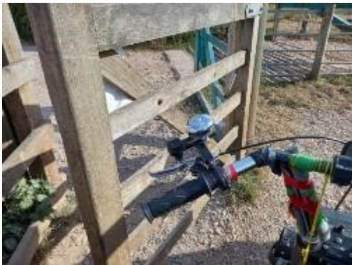
Photo 5. End gate at Countess Wear car park near Bridge Road.
