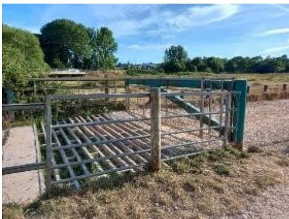
Photo 6. End gate at Countess Wear car park. No mobility scooter access.
