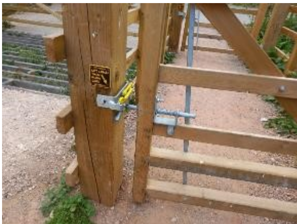
Photo 2. Centrewire easy latch system which is good for mobility scooter users.
